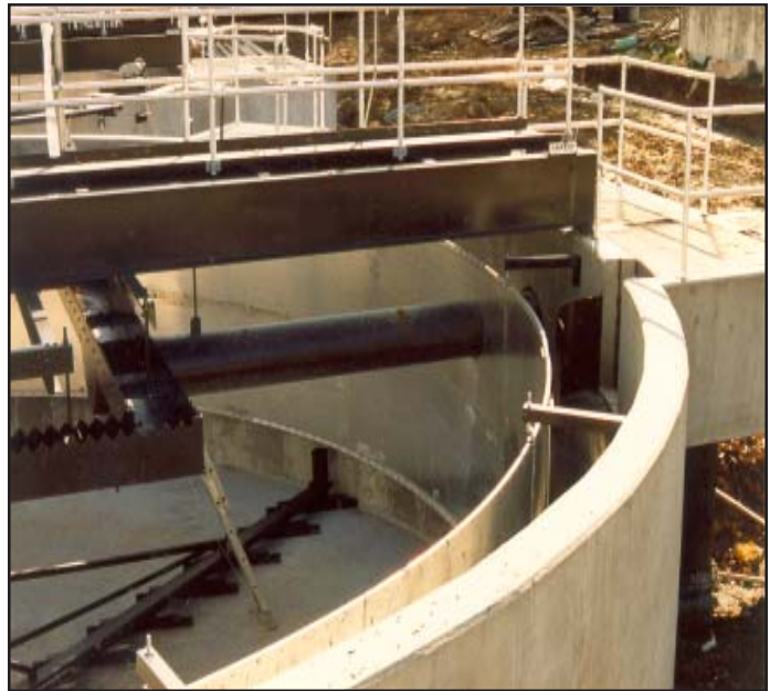
The influent and effluent pipes are conveniently located at the periphery of the tank for ease in tank bypassing.
