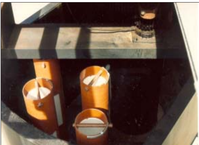
Smooth construction of the rotating valves reduces plugging problems and collection of stringy material.
