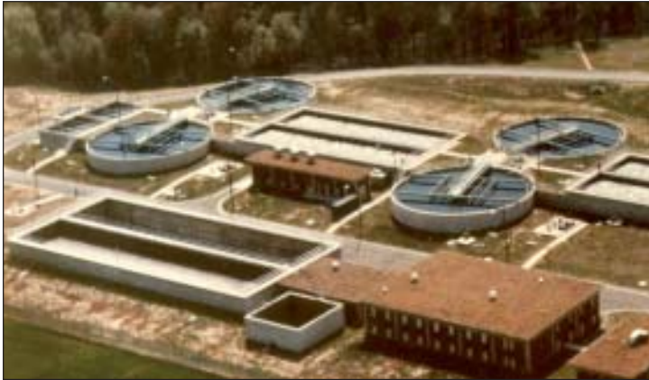
Dyersburg, TN • 2 - 75' Intermediate SPIRAVAC Clarifiers 2 - 75' Final SPIRAVAC Clarifiers
