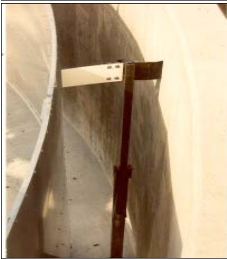
The hinged blade race skimmer enhances scum removal within the race area.
