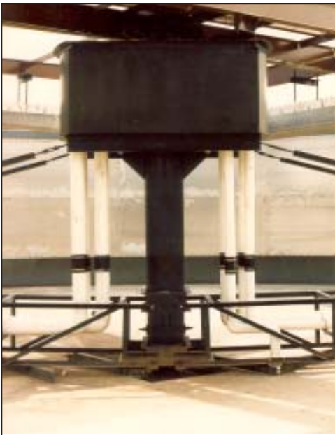
The suction sludge piping allows the operator to vary flow from each removal point within the center well.
